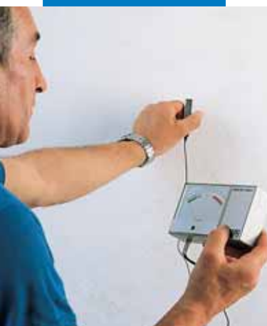
Checking plaster humidity
