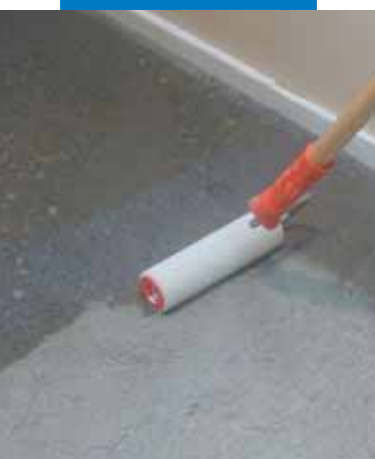
Applying Primer G with a roller
