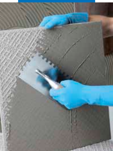
Spreading adhesive on the back of the tile
