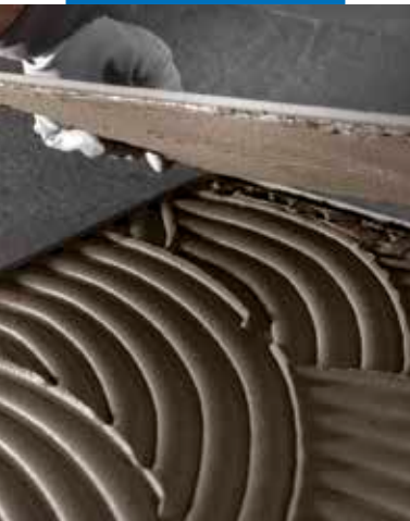
Installing thin porcelain tile on floor
