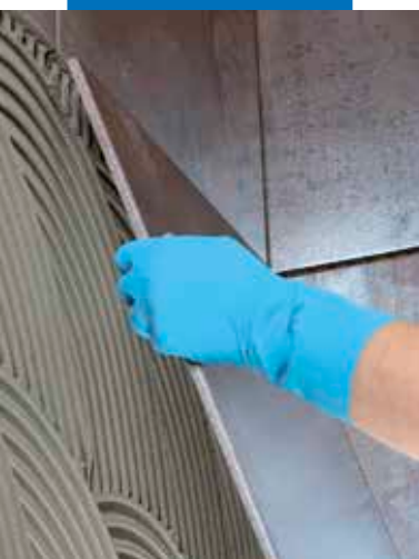
Laying large-sized tiles on walls
