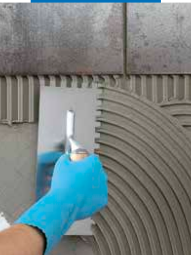
Spreading Ultralite S1 with a notched trowel on wall
