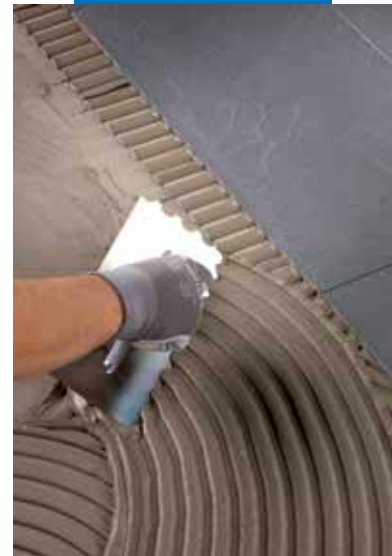
Spreading the adhesive on floor with a 9 mm round-tooth notched trowel
