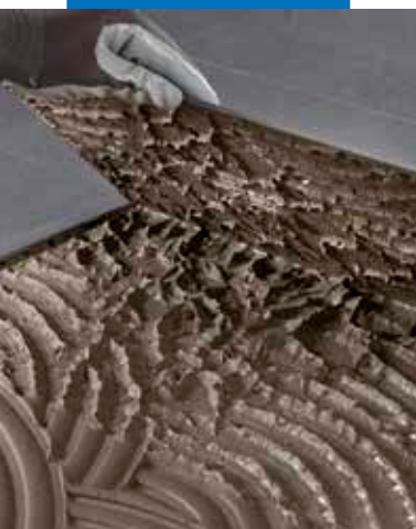
Checking the complete back-buttering of thin porcelain tile
