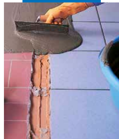
Smoothing existing flooring with Adesilex P4
