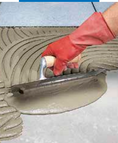
Spreading with semicircular notched trowel
