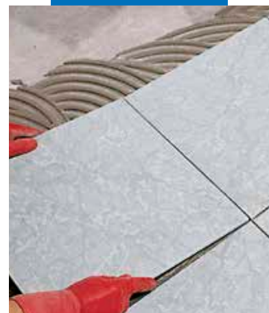
Laying porcelain tiles
