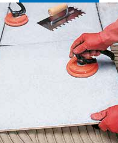
Laying large size tiles
